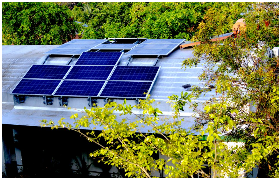
A 5.25 kW Solar System on the roof of a cottage ■ JGK and exported.
