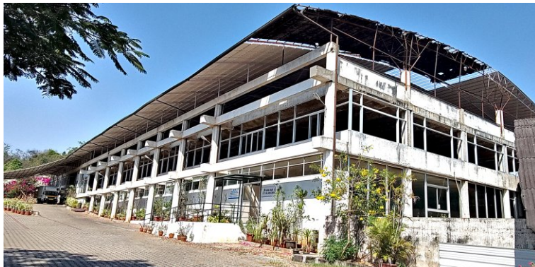
Renovation of the roof of Club House with white synthetic roofing sheets
