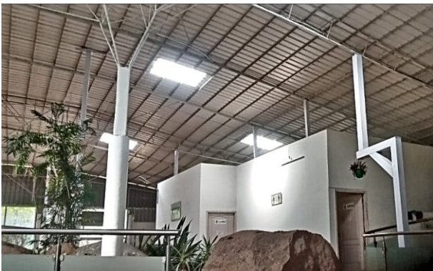
Additional structural support to reinforce the refurbished roof of the Club House
