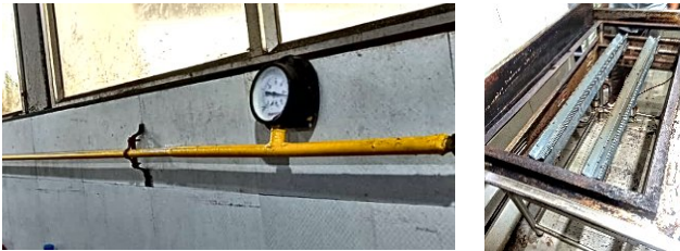
New gas plumbing and burners in kitchen
